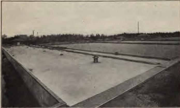
FILTER BEDS OF THE INDIANAPOLIS WATER WORKS.
